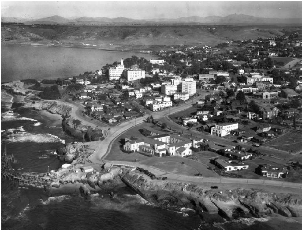
View of La Jolla showing the Children's Pool under construction, ca. 1931. ©SDHS, #90:18138-444-
